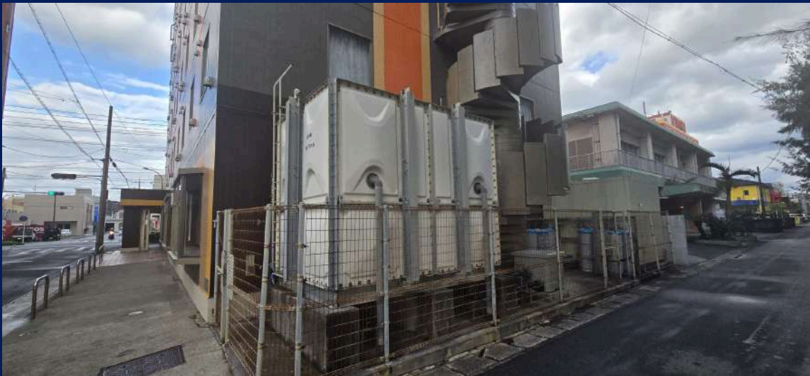
GRP (CTP) panel su deposu — saha montajı / GRP panel water tank, site assembly
