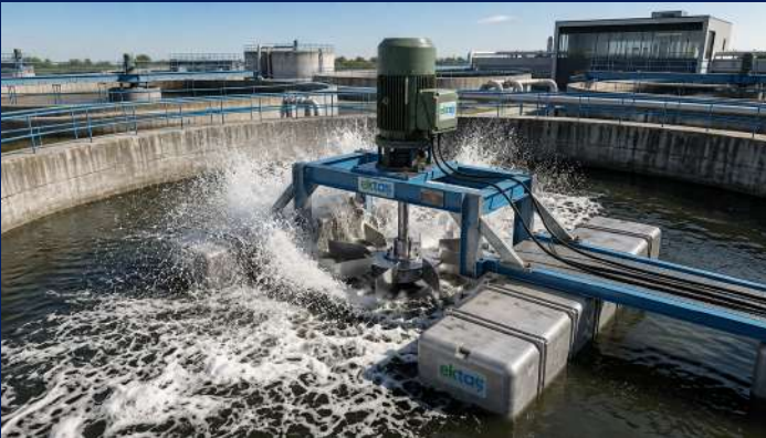
Köprü tipi yüzey aeratörü — dairesel havuz / bridge-mounted surface aerator, circular basin
